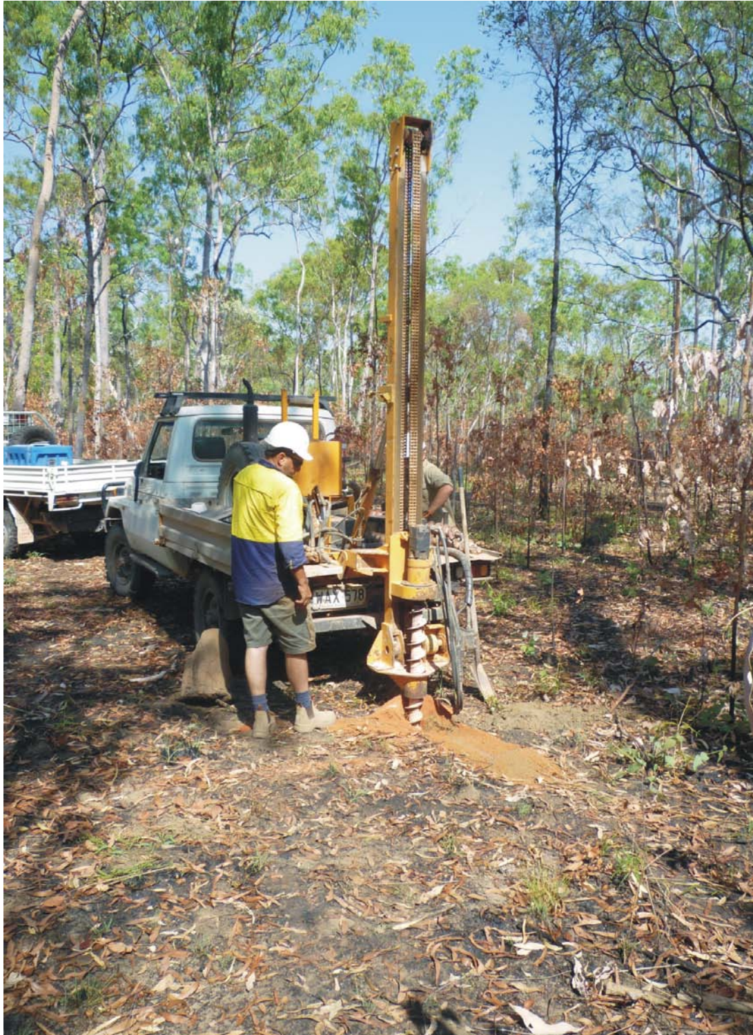
Plate 2: Auger drilling at Pretender Creek project.
